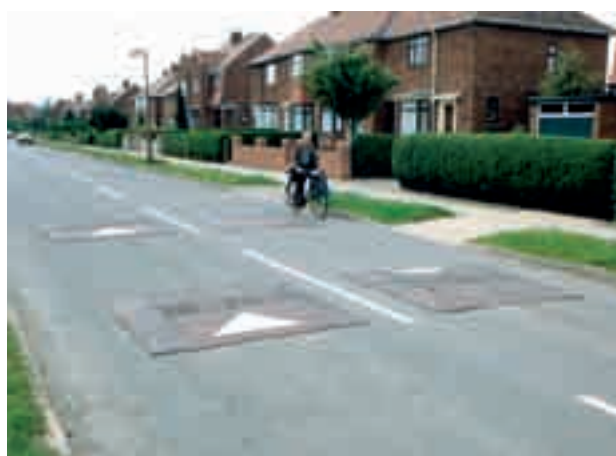
Fig 4.15 Speed cushions (left to right: two abreast, three abreast and double pair)
