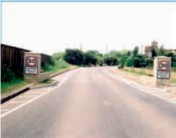
Fig. 3.8 Gateway feature, Latton
