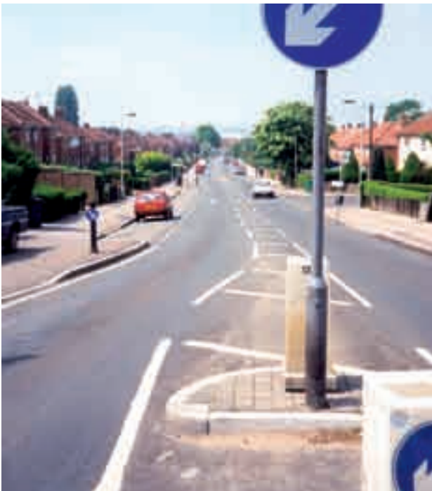
Fig. 2.5 Chicane of pedestrian refuge and sheltered parking
