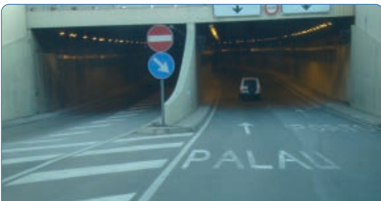
Road safety issues in Italy. In the first picture the landscaping restricts visibility between merging vehicles, in the second pedestrians are exposed to risk due to an absence of facilities, and in the third there is a risk of occupant injury from loss of control collisions with the wall. Photo source: Raimondo Polidoro
