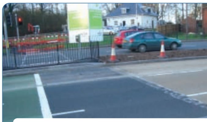
New set of traffic signals on a major development site
