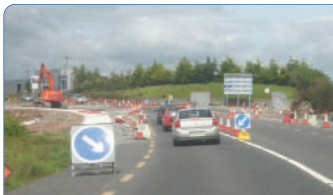
Road works in Ireland
