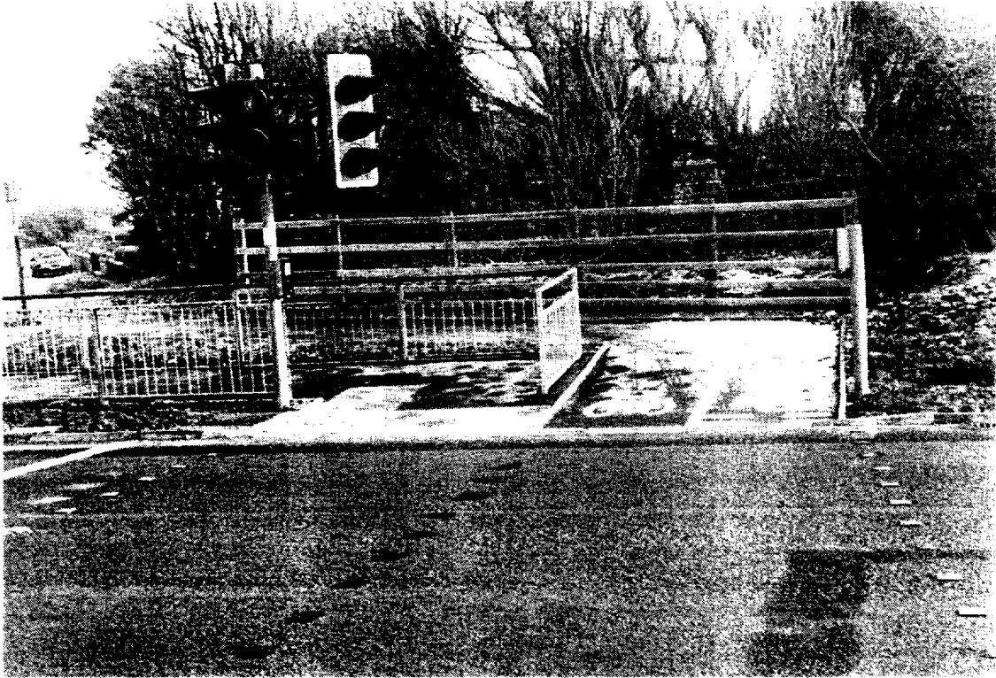
Plate 7 Cleveleys, nr Blackpool: A585(T) Amounderness Way/Linden Avenue (Lancashire County Council and North West Regional Office, DOT)
