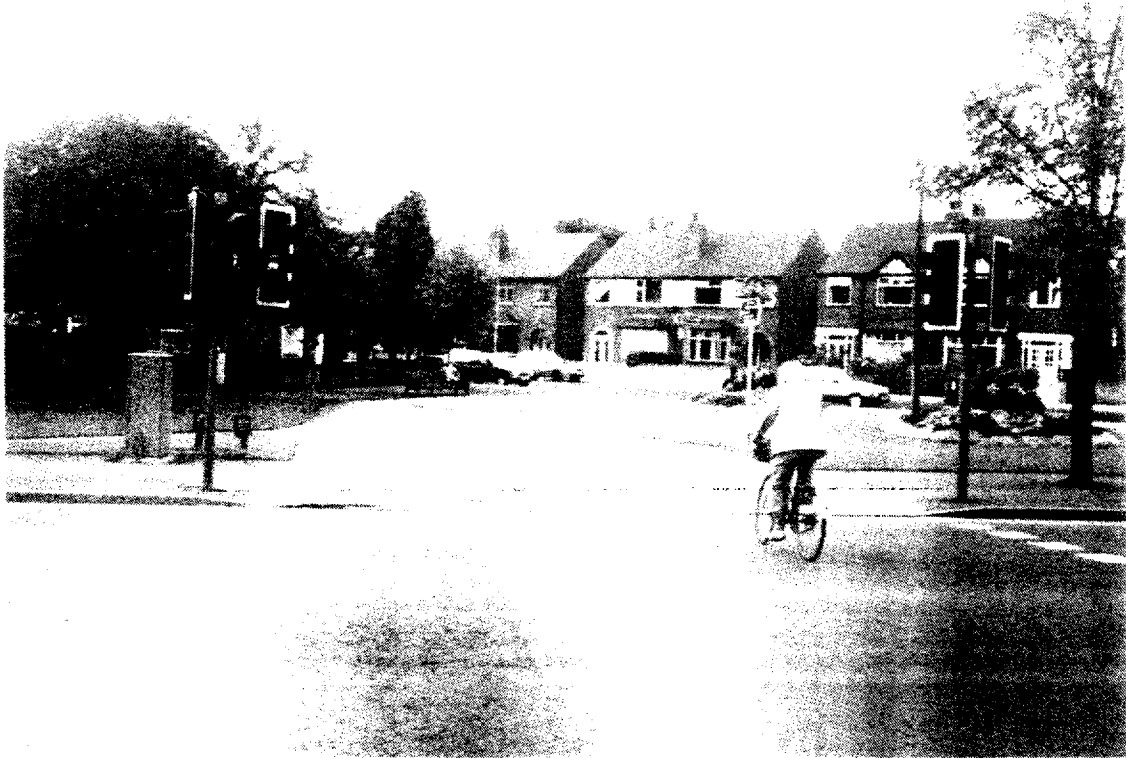
Plate 8 Nottingham: Queens Road, Beeston (Nottinghamshire County Council)
