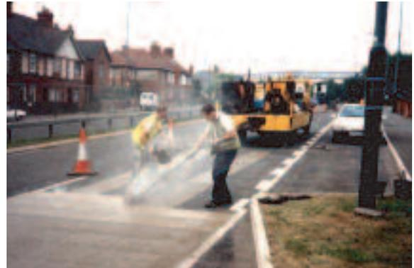
High-friction or 'anti-skid' surfacings are surfacings that make use of aggregates with better skid-resistance properties than normal, generally an artificial aggregate produced out of the "residue" from aluminium called calcined bauxite. In order for the aggregate to be retained on the surface with the high stresses expected, the binder needs to be stronger than can generally be achieved with conventional materials.
